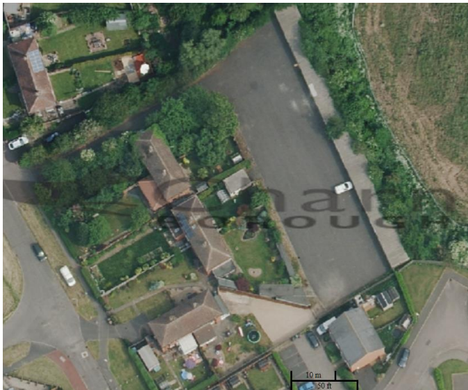
Figure 6 - Site at Manor Road, Loughborough
